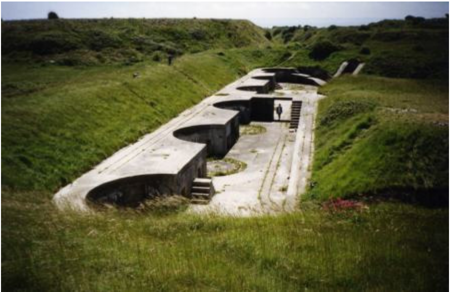
Remains of the high angle battery on Portland
